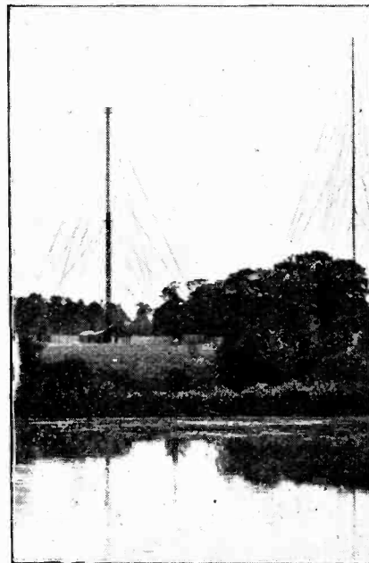
BURNT DOWN. A general view of the Ditton Park Radio Research Station which suffered severe damage in a fire last week. The mast on the right was burnt to the ground.
